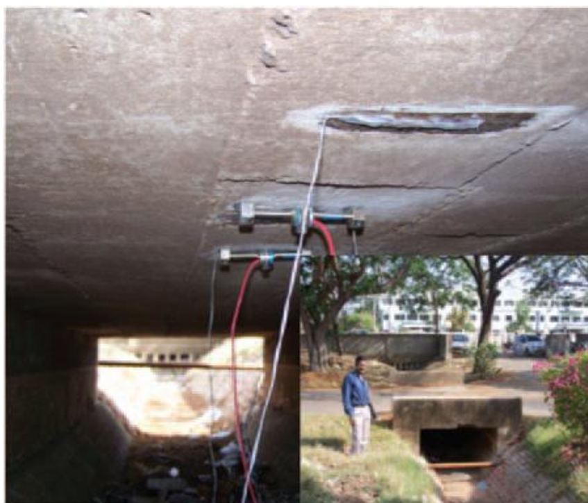
FIG 4(b) INSTRUMENTED CULVERT
