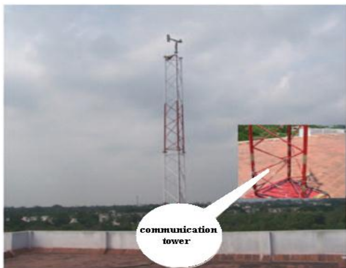
FIG 4(a) INSTRUMENTED COMMUNICATION TOWER
