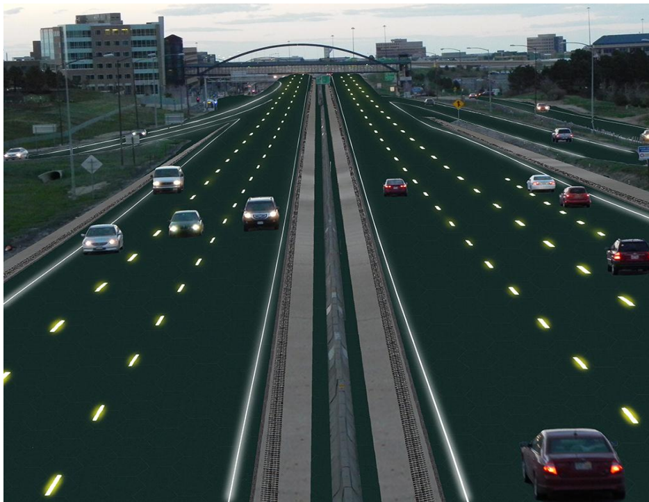
Figure 3. Smart Illuminated Roadway
