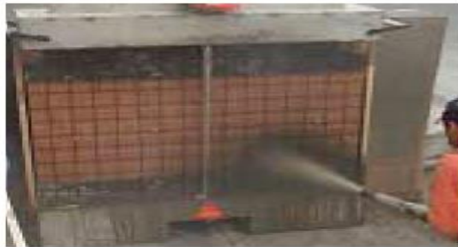
Fig3-shotcrete method.
