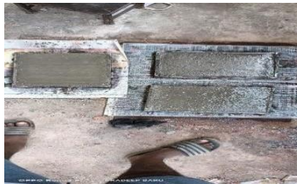
Fig 3.3 forming of tiles
